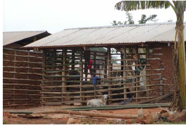
Fig.19 Wattle & Daub house under construction at Yaayaaso
